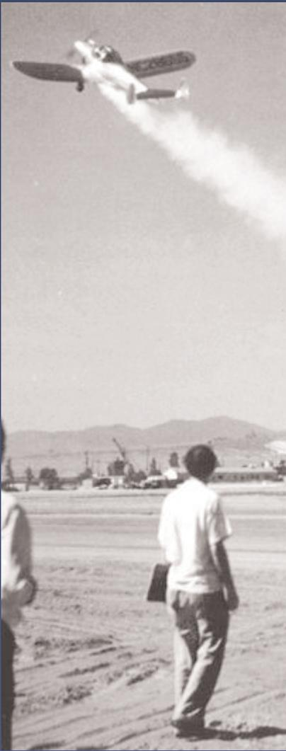
**Take-off of America's first "rocket-assisted" airplane, an Ercoupe fitted with a GALCIT developed solid propellant 28 pound thrust JATO (Jet Assisted Take-Off) booster. The Ercoupe took off from March Field, California and was piloted by Captain Homer A. Boushey Jr.**
