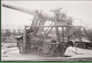
Fort Hancock installed the nation's first "disappearing gun" battery in 1893. After firing, the carriage retracted down into a bunker, keeping it out of sight of an enemy while it was being reloaded. While effective, the mechanism was complex and by the 1920s the design was withdrawn from active service.
